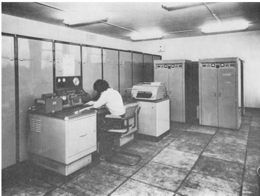
Plate IV. Mercury computer at Meteorological Office Headquarters, Bracknell, showing console and magnetic drums.
