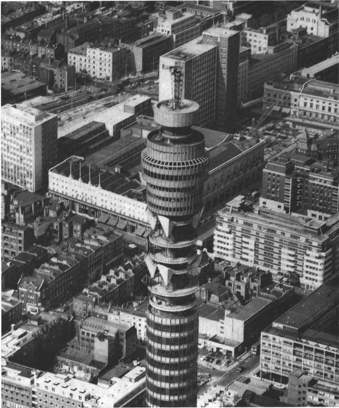
An aerial view of the GPO Tower showing the weather radar installation. This is a Plessey 42A Weather Radar and is to be seen at the top of the 40-foot lattice mast.
