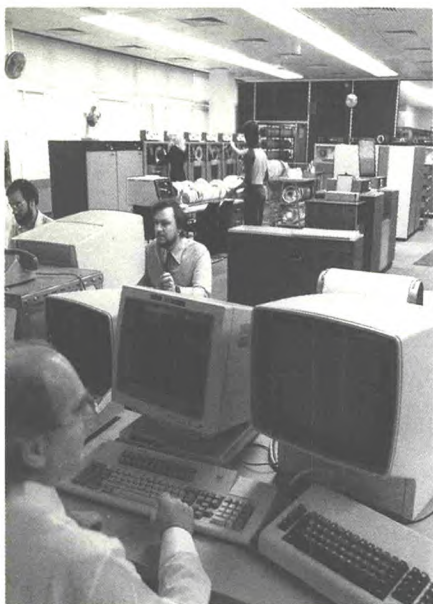
The operators' consoles and magnetic tape units in the COSMOS computer room. Part of the primary tape library can be seen in the background.
