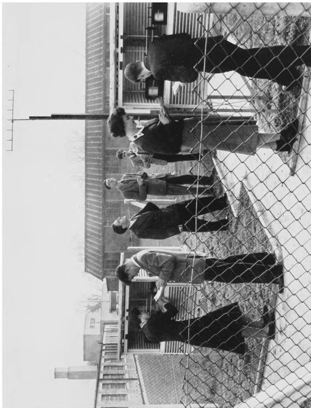
METEOROLOGICAL OFFICE TRAINING SCHOOL Assistants taking the readings in the instrument enclosure
