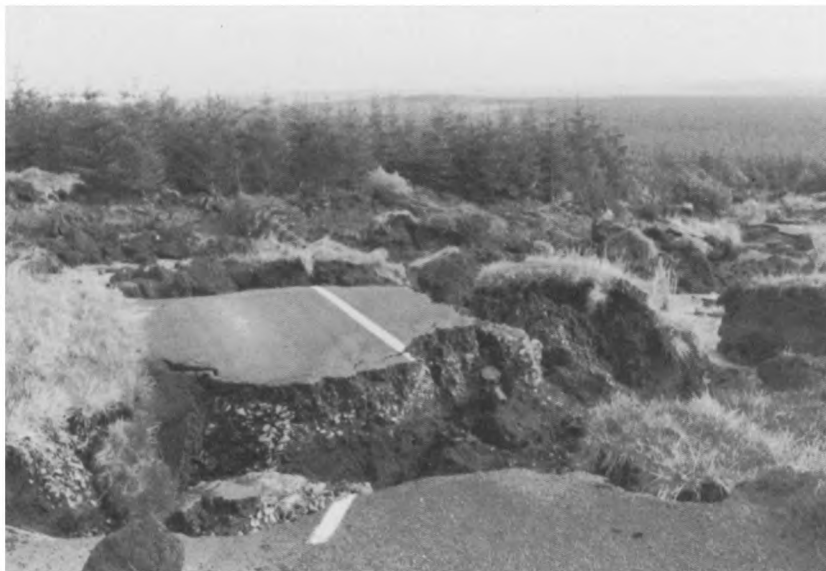
Plate III. Section of road hurled some 200 to 400 metres down the hillside at Orra Beg on 1 August 1980.
