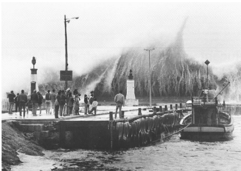
The picture above, kindly donated by The Argus shows a wave breaking over the Kalk Bay harbour wall. Damage to the breakwater later allowed the waves to get into the harbour itself, and this led to the destruction of the wooden quay in the foreground.
