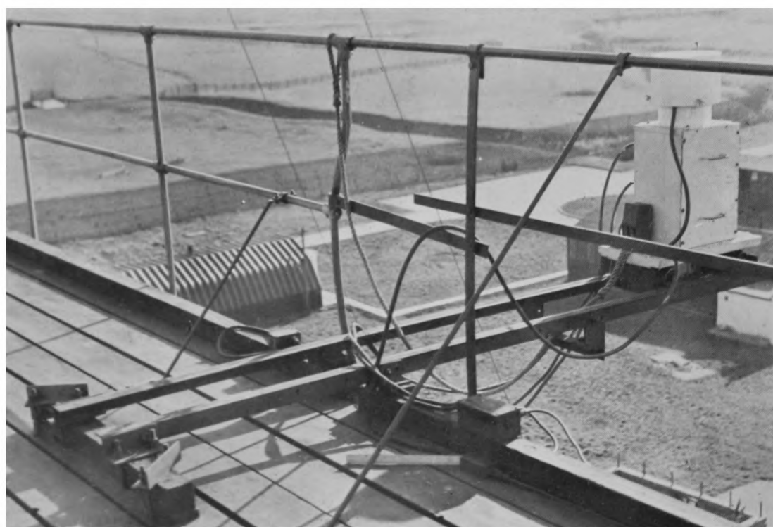
FIG. 3- DEVICE FOR RETRACTION OF SCREEN
