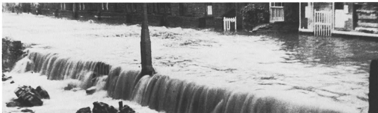
Figure 5. Flood-water flowing down the Halifax Road, Cullingworth, on the evening of 11 June 1956, causing severe damage in houses and breaking down 36 metres of the wall along the road The Yorkshire Observer .
