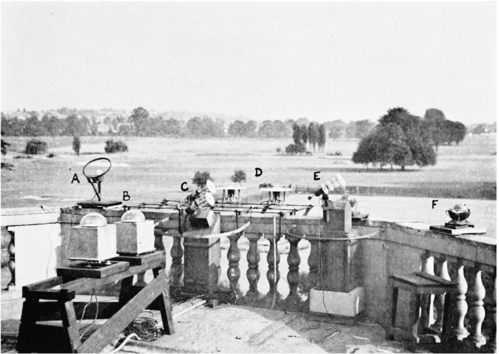
PLATE I—SOLAR RADIATION EQUIPMENT AT KEW OBSERVATORY, 1953
