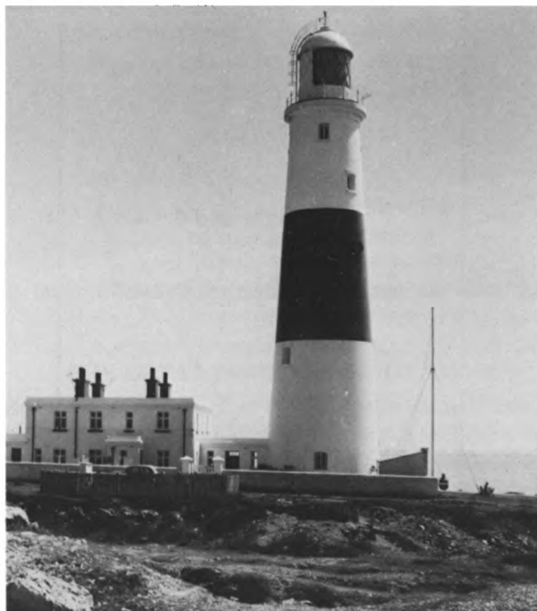
Figure 4. Electrical anemometer head and vane on top of the lighthouse. The exterior ladder allows access for servicing.
