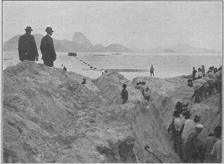
Cable being landed from lighter, the cable ship not being able to approach the cable landing owing to shoal water.
