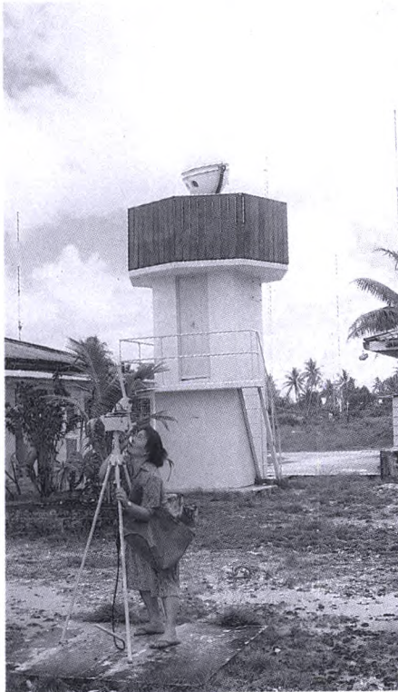
WWW in operation — Funafuti, Tuvalu, Pacific Ocean. A balloon carrying a radar target is being followed visually just after launch to allow the Plessey WF3 radar (white sphere) to follow it automatically. Winds to stratospheric heights are measured twice daily. Replacement of the radar with the more modern WF33 is in hand.
