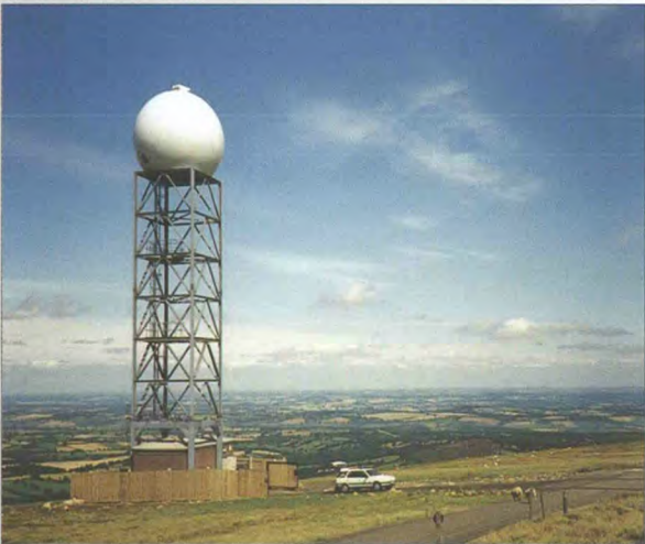
A new rainfall radar at Clee Hill in Shropshire entered service in September 1993. This radar can measure wind fields within rain areas and the vertical extent of the rain cells.
