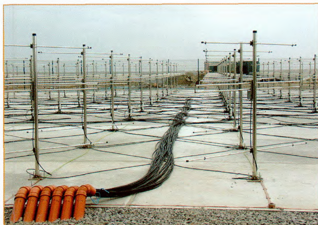
Figure 3. Antenna installation for 64 MHz tropospheric wind profiler on South Uist.
