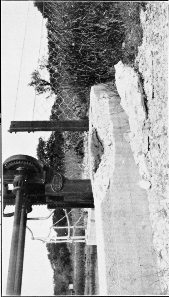
FLOOD-GATE ON THE RIVER PIDDLER, WAREHAM, DAMAGED BY LIGHTNING, MAY 25TH—26TH, 1937.
