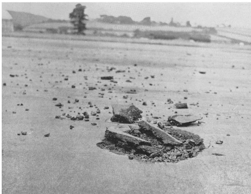
PLATE V—DEBRIS FANNING OUT FROM THE CRATER FORMED BY THE LIGHTNING STRIKE AT CHIVENOR
