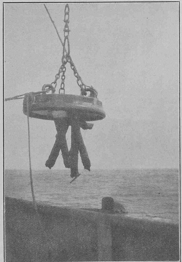
Salving pig iron from a wreck with an electric magnet.
