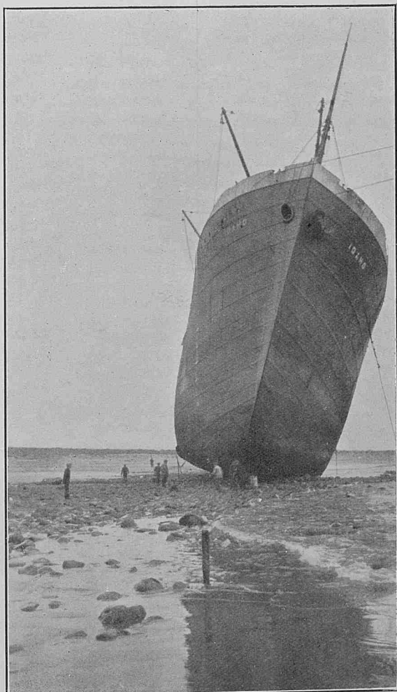
The S.S. Idaho high and dry. Owing to shortage of water and the vessel's lack of stability when empty she proved a difficult case for refloating, very heavy ground tackle had to be laid out, and heavy purchases worked from either side of the vessel to keep her upright until she was drawn into sufficiently deep water to permit of water ballast being used.
