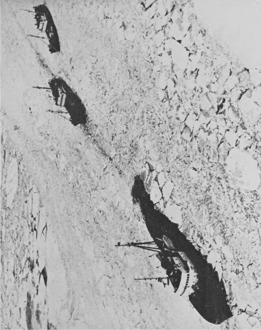
PLATE I—A SWEDISH ICEBREAKER CLEARING A PASSAGE FOR TWO FISHING VESSELS THROUGH THE FROZEN SEA OFF MALMÖ IN FEBRUARY 1963
