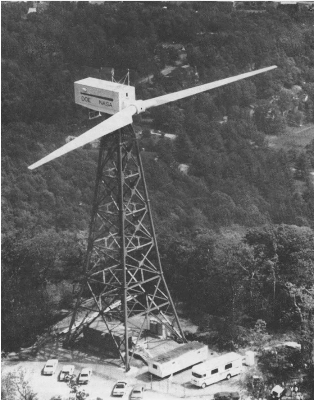
Plate I. Two-hundred foot diameter wind turbine rated at 2 MW. Completed in summer 1979 at Boone, North Carolina. Constructors General Electric Co. Blades by Boeing Engineering and Construction.
