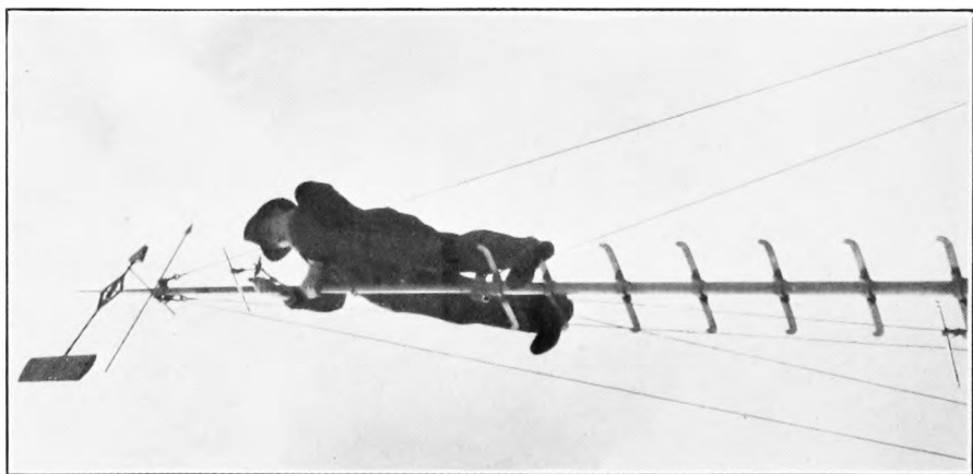
FIG. 1 (a).—WIND VANE MAST WITH 10 FT. AND 20 FT. THERMOMETERS
