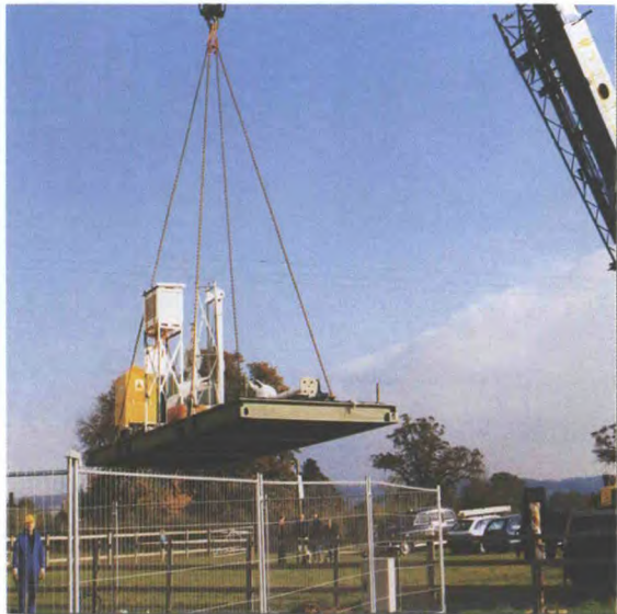
Mobile Semi-Automatic Met. Observing System being installed at Coleshill (near Birmingham Airport)
