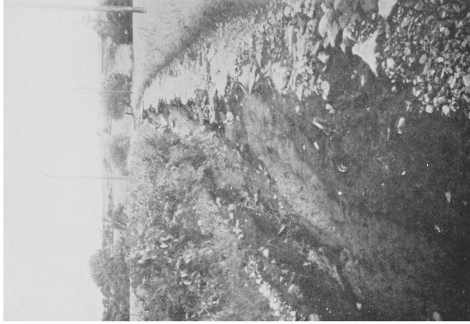
GULLY ERODED IN ROAD TO TOR-Y-FRON FARM The road had a macadamized surface over consolidated ash.
