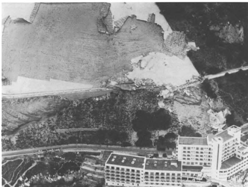
Figure 5. Damage to east-facing water catchments at Gibraltar, March 1975.
