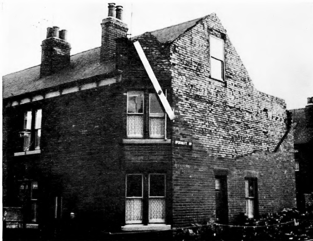
Reproduced by permission of the City Engineer, Sheffield PLATE I—STRIPPING OF OUTER WALL OF A CORNER HOUSE
